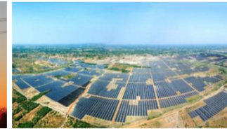
648 MW Ultra Mega Solar Power Plant
