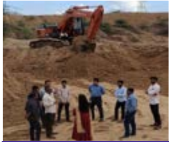
Restrengthening & Desilting of Check dam – 720+ Benefited
