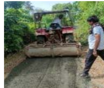
Renovation of Approach road Vadi Vistar at Mota bhadiya village.- 7200 Benefited
