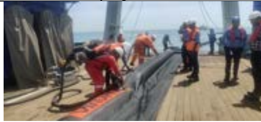
Boom laying from Dol 11
