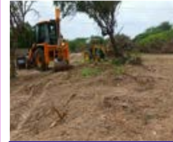
River Cleaning and JCB Support - 2250+ Benefited
