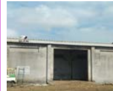
3 Villages - Renovation of Godown and Gauthala Shed
