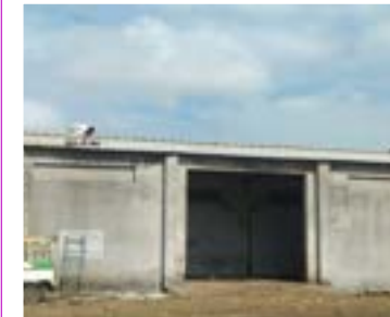
3 Villages - Renovation of Godown and Gauthala Shed
