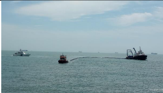
J formtion making in progress
