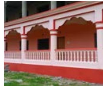
Renovation of High School at Zaarapa – 2200+ Benefited
