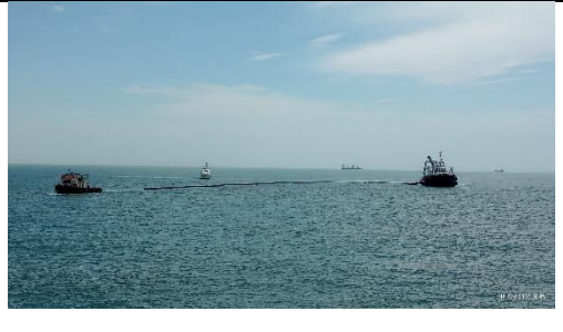
J formtion making in progress
