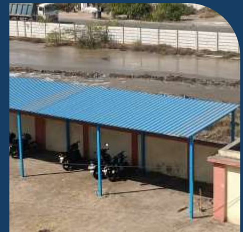
Renovation of Civil and Electrical Work at ITI, Mundra - 500 students benefited
