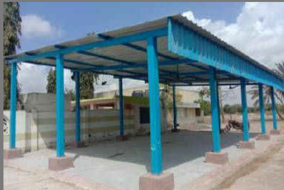
Construction of Shed at BRC Bhavan
