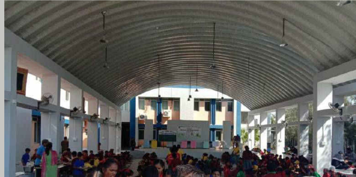
Construction of Prayer Shed at AVMB
