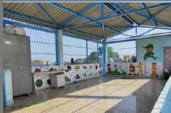
Upgradation of Balwadi at Zarpara
