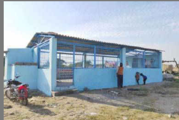
Renovation Balwadi at Bavdi Banadar
