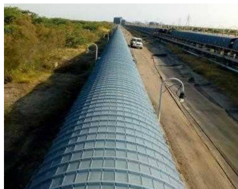
Closed Conveyor System
