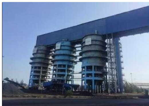
Closed Silos for Truck & Wagon Loading
