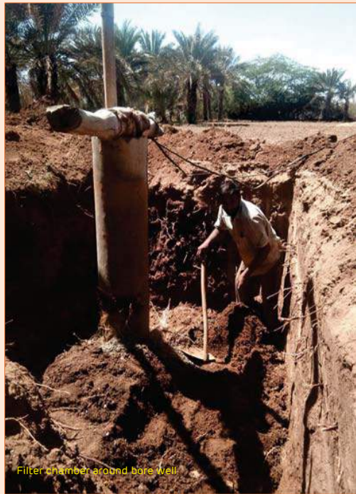
Min filter chamber for bore well
