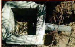
Min filter chamber for bore well
