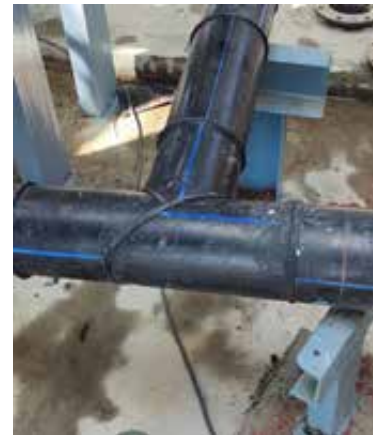
HDPE pipeline repairing miscellaneous jobs
