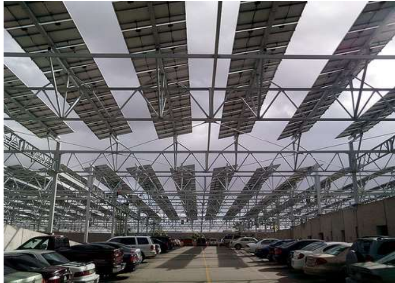
Figure 52 Solar Panel Installation on Parking Shed
