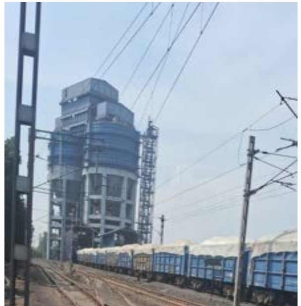
Silo Facility with teliscopic chute system
