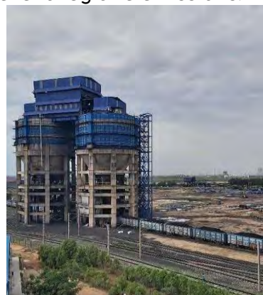
Silo Facility with teloscopic chute system
