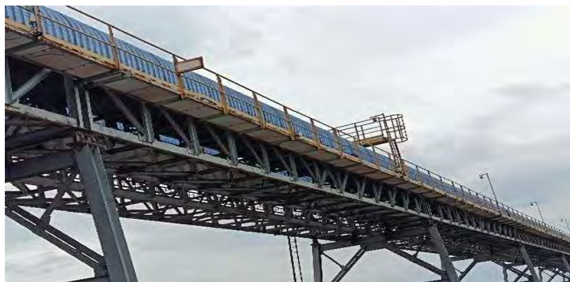
Grab ship unloaders and Hoppers, discharge/feeding points
