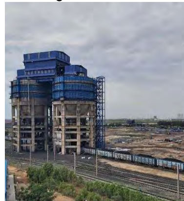
Silo Facility with teloscopic chute system
