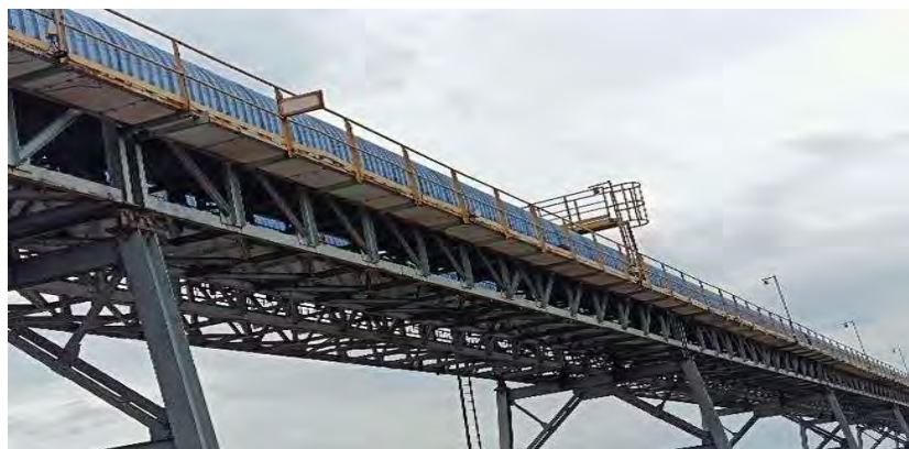
Grab ship unloaders and Hoppers, discharge/feeding points
