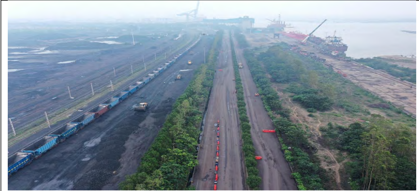
Green Belt – Coal sidings
