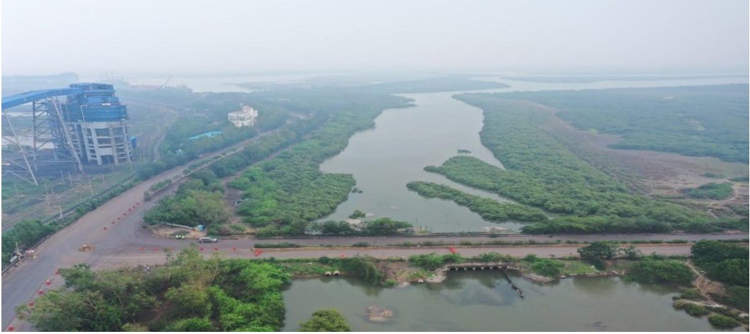
Greenbelt Protection to Buckingham Canal inside the port premises
