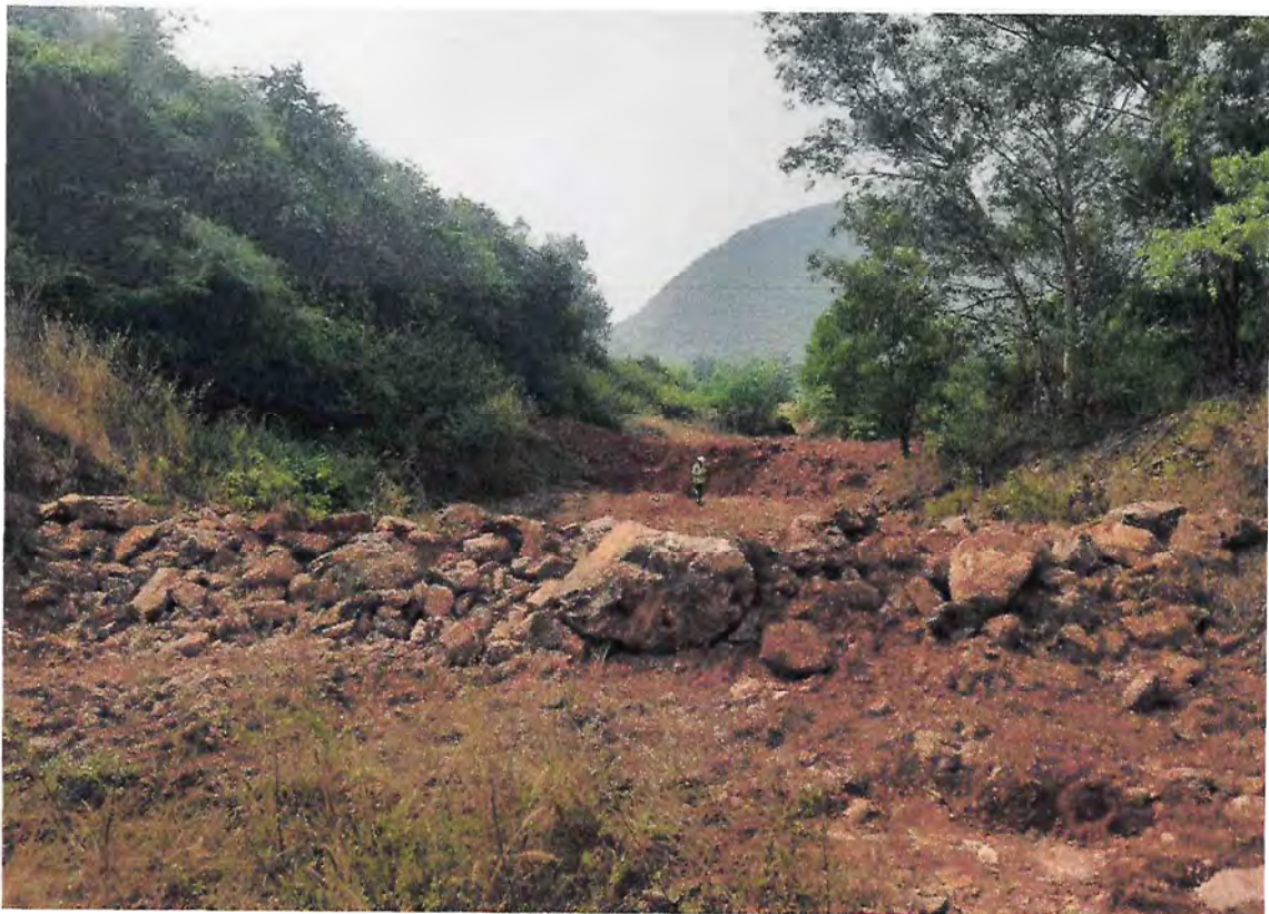
Retaining wall followed by trench
