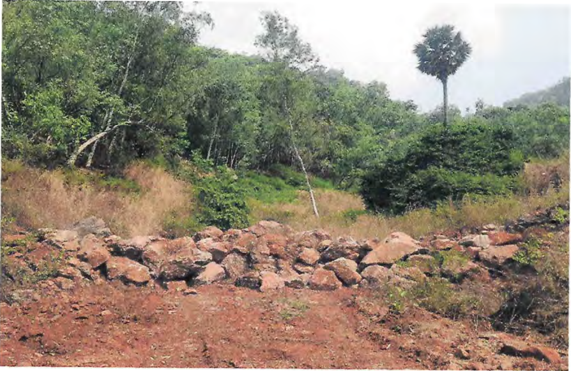
Greenbelt followed by Retaining wall
