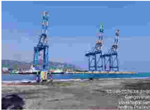
Container handling equipment
