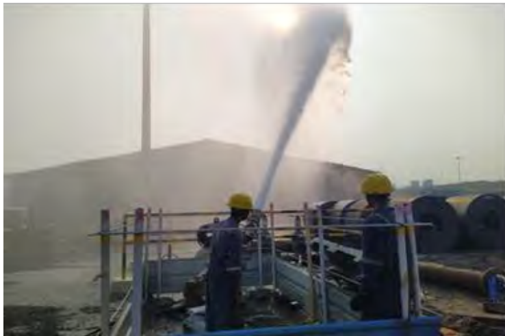
Water hydrant line with fire tower and hose reel points installed at Jetty area. Regular mock drills on fire fighting are being conducted.
