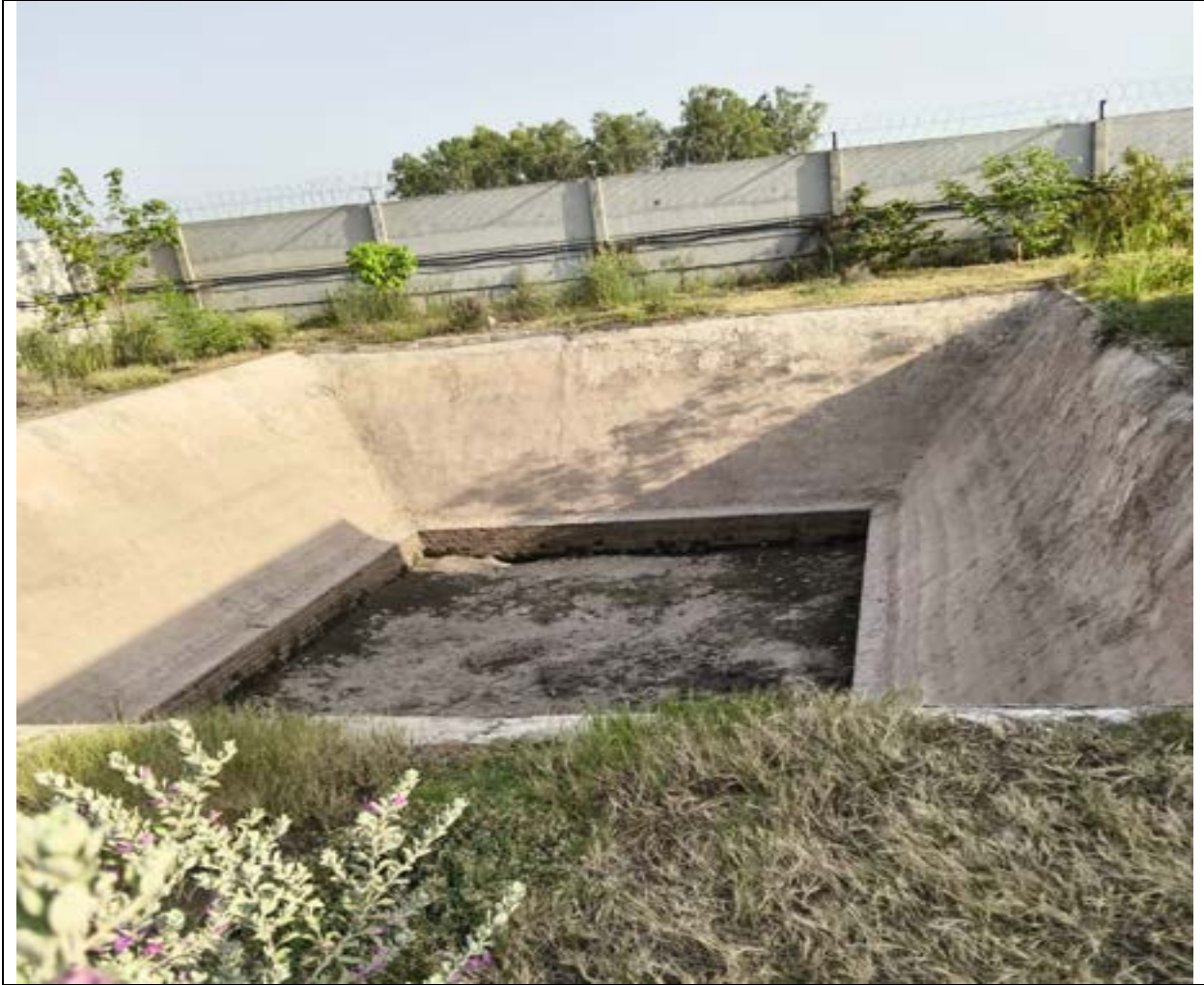
Rainwater Harvesting Structures
