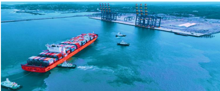
Vizhinjam: India's first automated port
