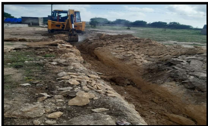
Digging activities for pipeline laying at village - Rampar
