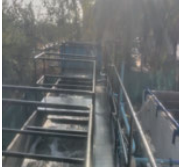
Aeration and plastic media plate form replacement work has been completed at Adani house STP
