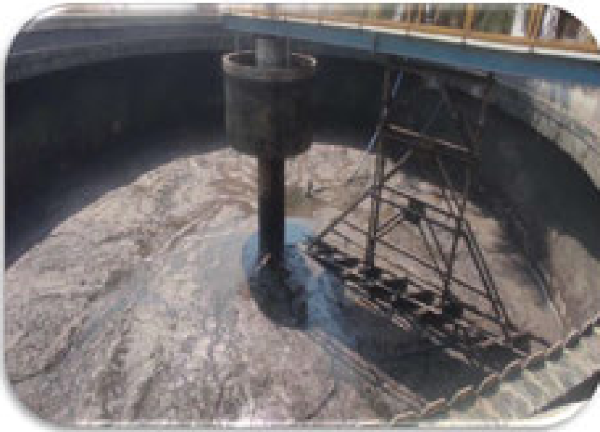
Secondary clarifier 1 and chlorination tank cleaning work
