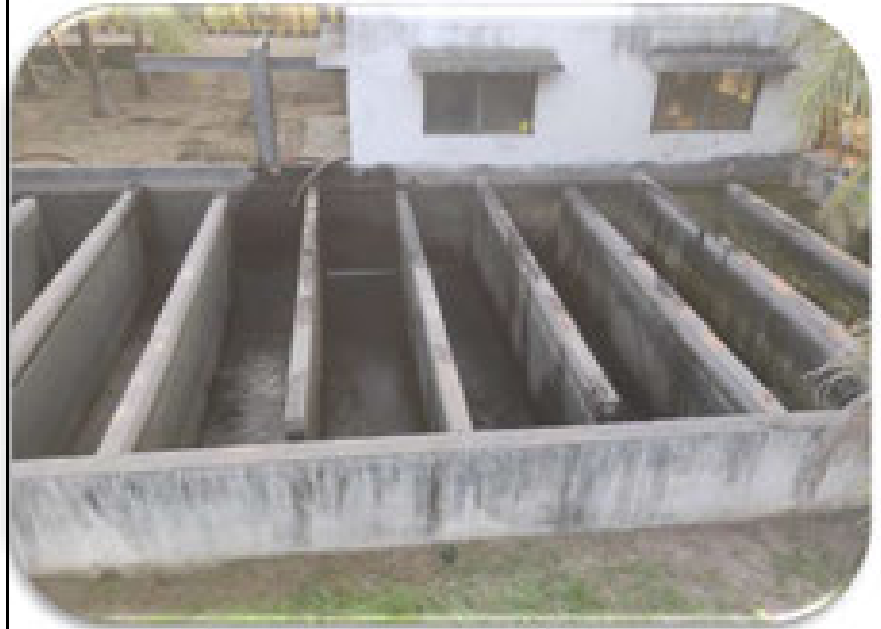
Secondary clarifier 1 and chlorination tank cleaning work
