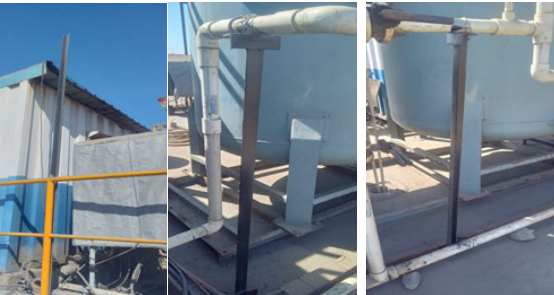
Pipe supports and light support angle installation work has been done
