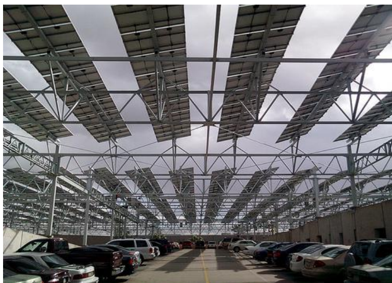
Figure 85 Solar Panel Installation on Parking Shed
