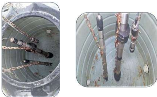
Cleaning work of CETP online analyzer tank and sensor
