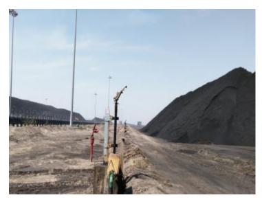
Adequate distance between two heaps with fixed fire fighting & water sprinkling
