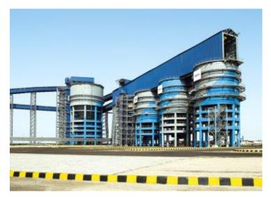
Mechanised Coal Handling System with closed conveying
