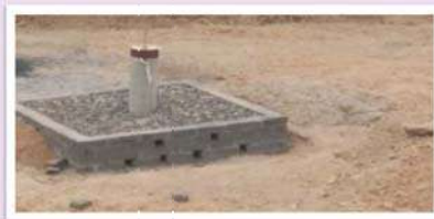
Mangara- Artificial bore well recharge – work completed
