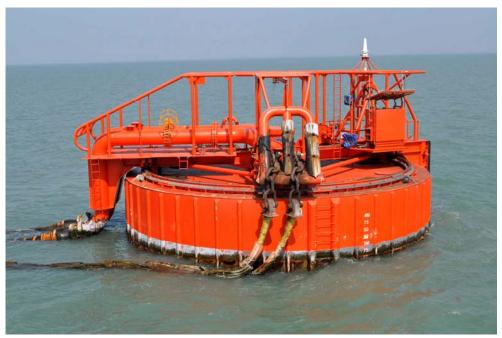
SPM, Crude Oil Terminal and Connecting Pipes
