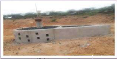
Borana- Artificial bore well recharge –work completed
