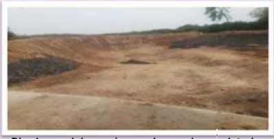
Dhrub- pond deepening work – work completed
