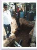
Mota Kapaya- abandoned bore well recharge – work completed
