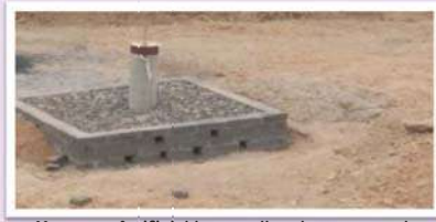
Mangara- Artificial bore well recharge – work completed
