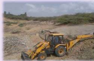
Zarpara- west weir repairing work
