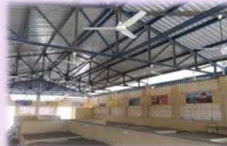
Driver Rest Shed at North Gate
