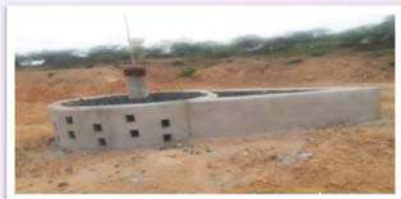
Borana- Artificial bore well recharge –work completed
