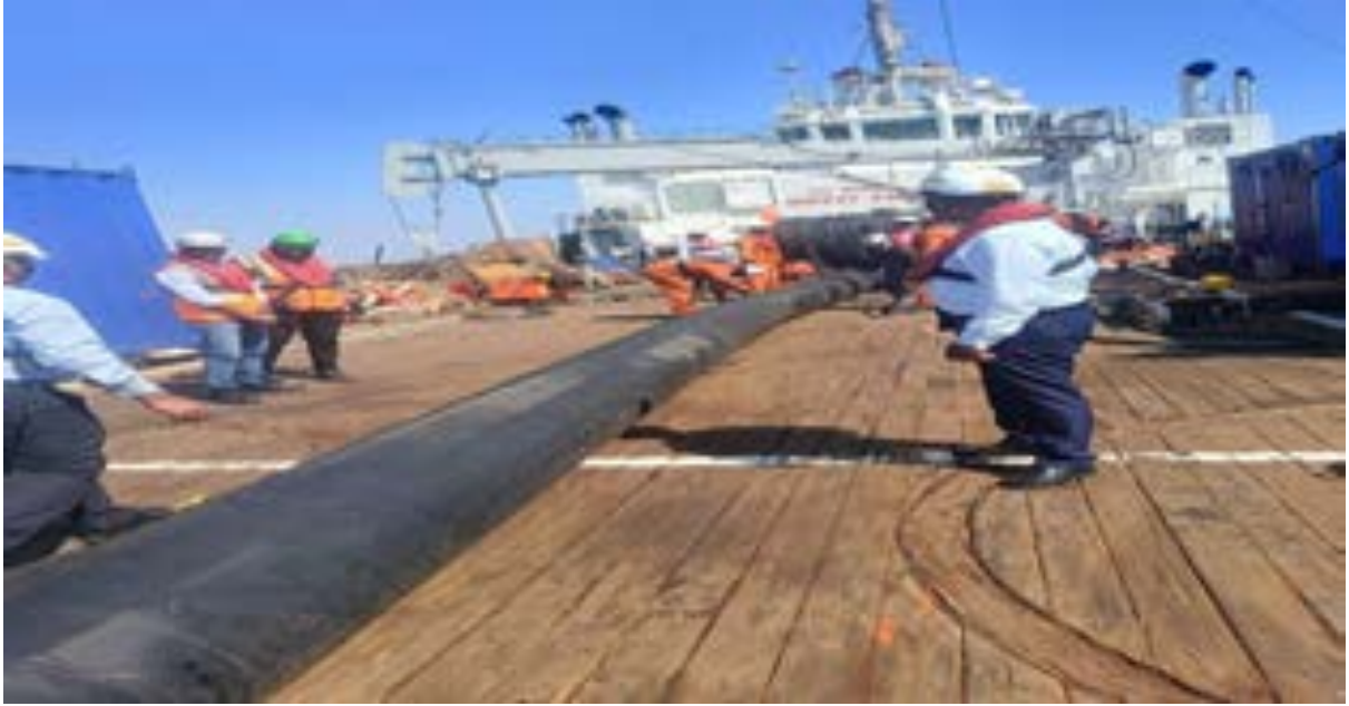
Boom laying from Tug Dol 11
