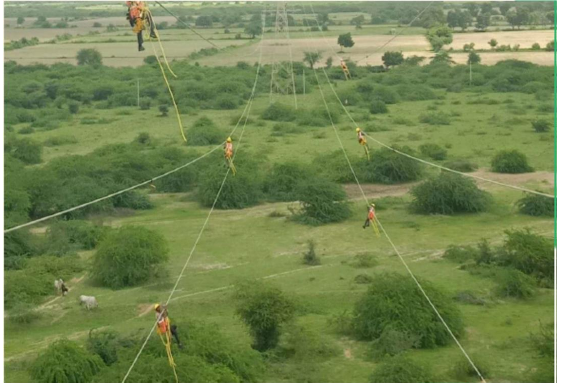
Installation done by trolley
