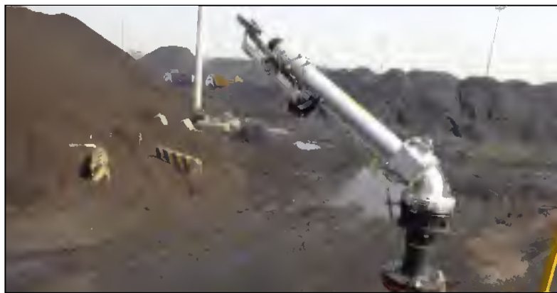
Water Sprinklers installed for Dust Suppression
