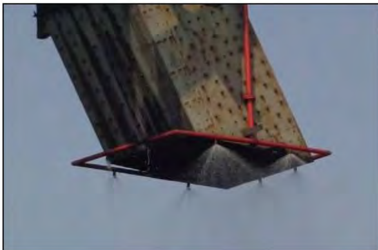
Coal Chute point having water Sprinkling System
