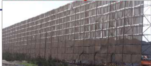
Wind Brake Shield At Coal Yard Area
