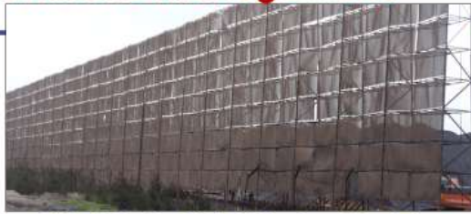
Wind Brake Shield At Coal Yard Area
