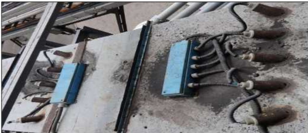
Dust Suppression System Installed in Conveyor System
