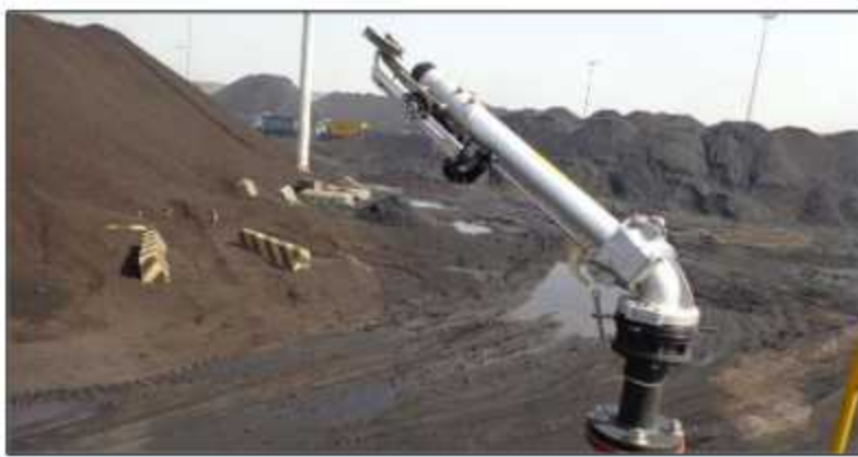
Water Sprinklers installed for Dust Suppression
