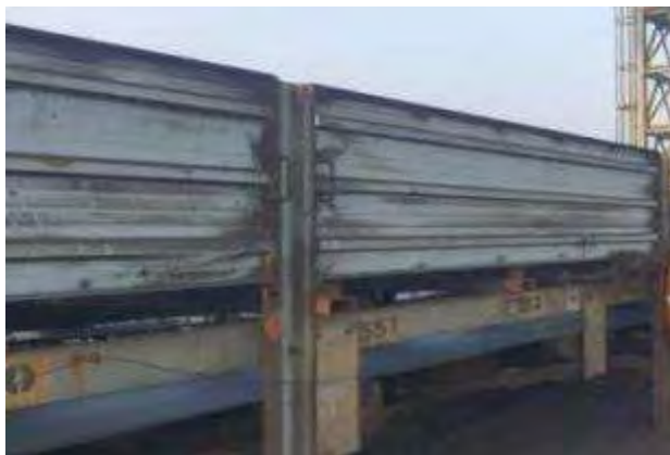
Cladding to conveyor belt
