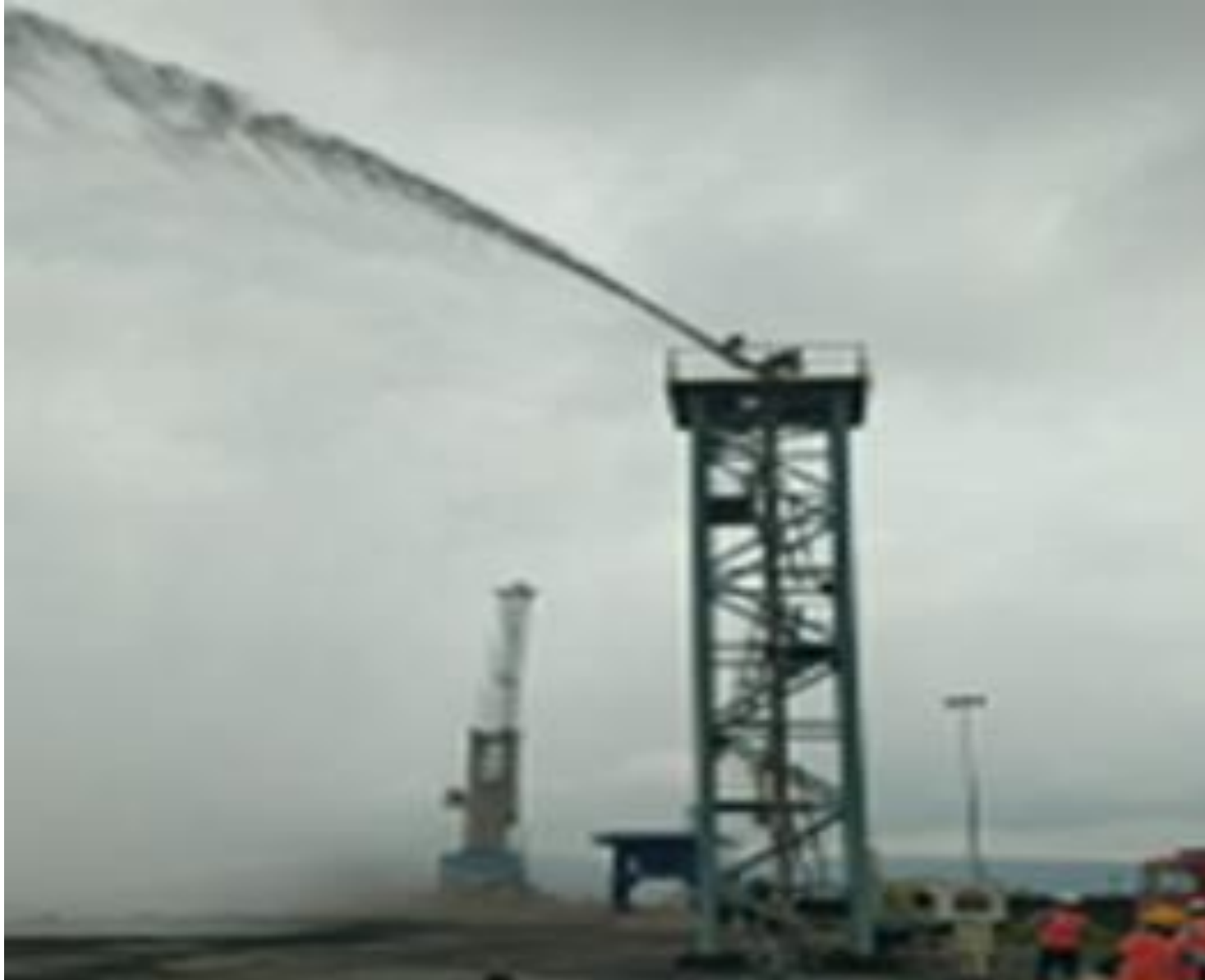
Water hydrant line with fire tower and hose reel points installed at Jetty area
