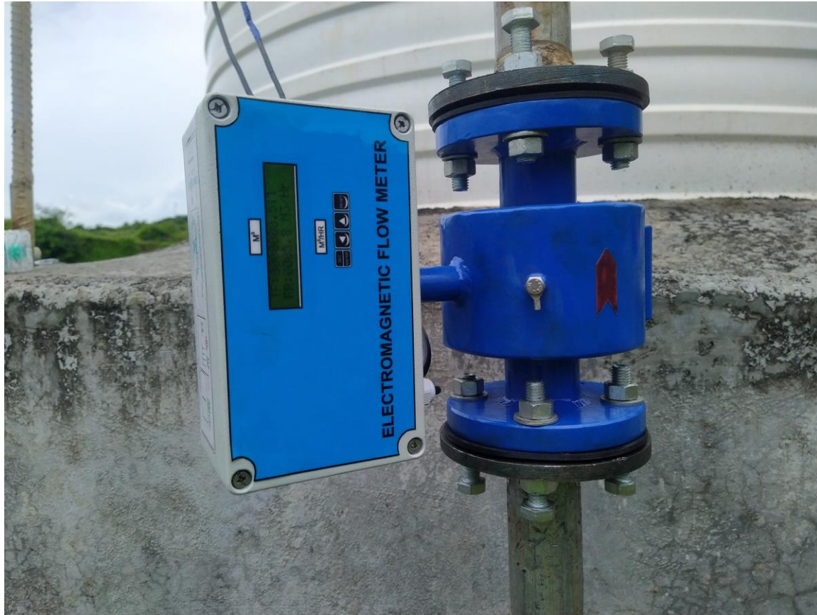
Installation of Flowmeter with telemetry
