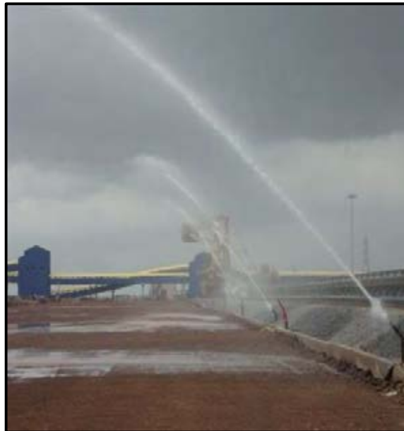
Rain Guns at Stack Yard
